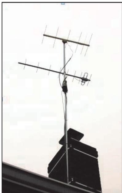
The smaller antennas, 1.25m and 70cm, were put on a rotator and strapped to the chimney. This was the first time I had ever used a rotator. Up to now, all of my rotating was done by me, which is ok, I don't mind the activity. However, it is next to impossible to peak a signal that way. Go outside, rotate a little, go back inside, check the radio, repeat. (I will have to acquire two more rotators...)
